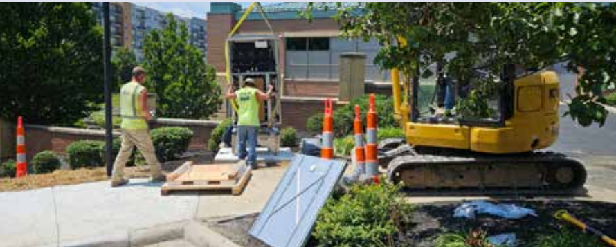
Anderson Center’s EV charging station is taking shape.
